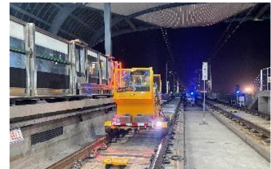
Hohhot Wuhai Works Section
